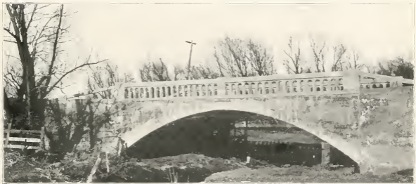
CONCRETE BRIDGE AT MALCOM
